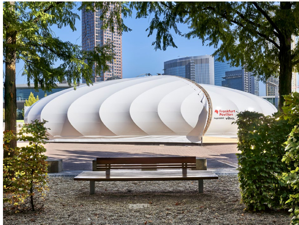
Frankfurt Pavilion temporary building Designer : schneider+Schumacher, Bollinger+Grohmann, Frankfurt / Main, DE
