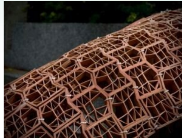
3D-printed ceramic bricks forming a double-curved masonry structure
